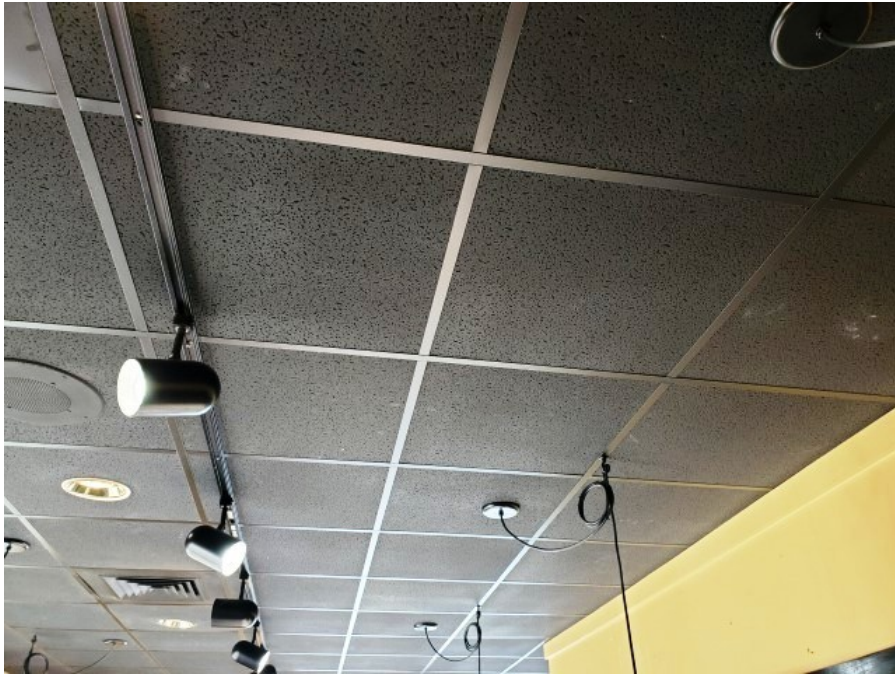
Photo 3: View of dining room ceiling tiles.
