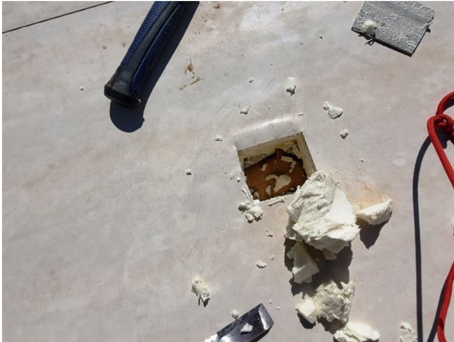
Photo 10: View of roof core sample, and wooden roof deck.
