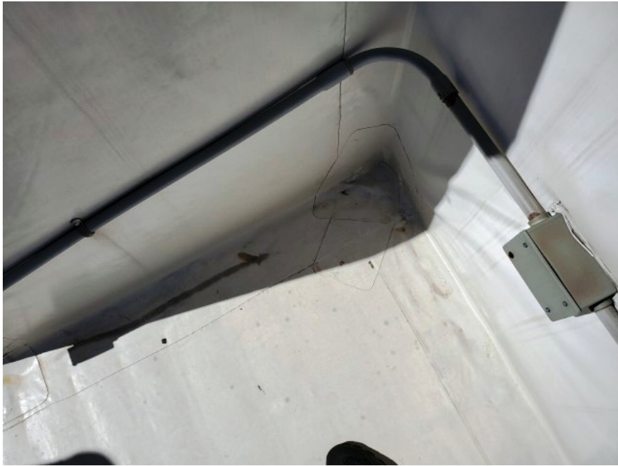
Photo 9: View of TPO flashing.
