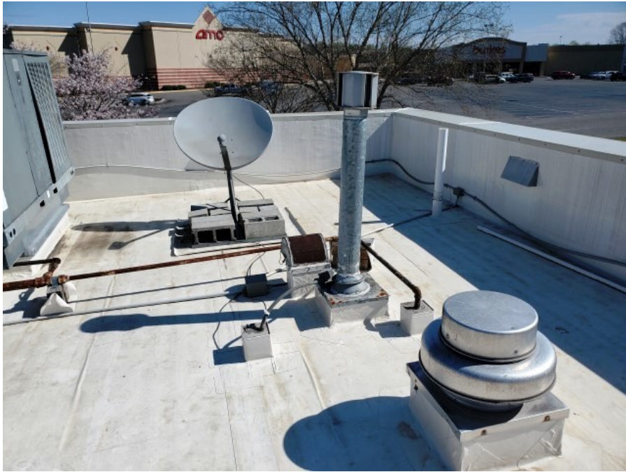
Photo 7: View of TPO roofing system.
