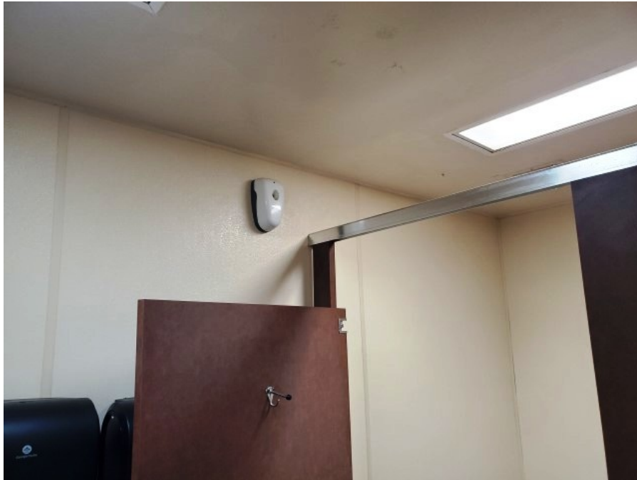
Photo 6: View of resilient wall panels and sheetrock ceiling.
