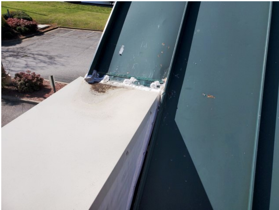
Photo 12: View of white roof caulking.
