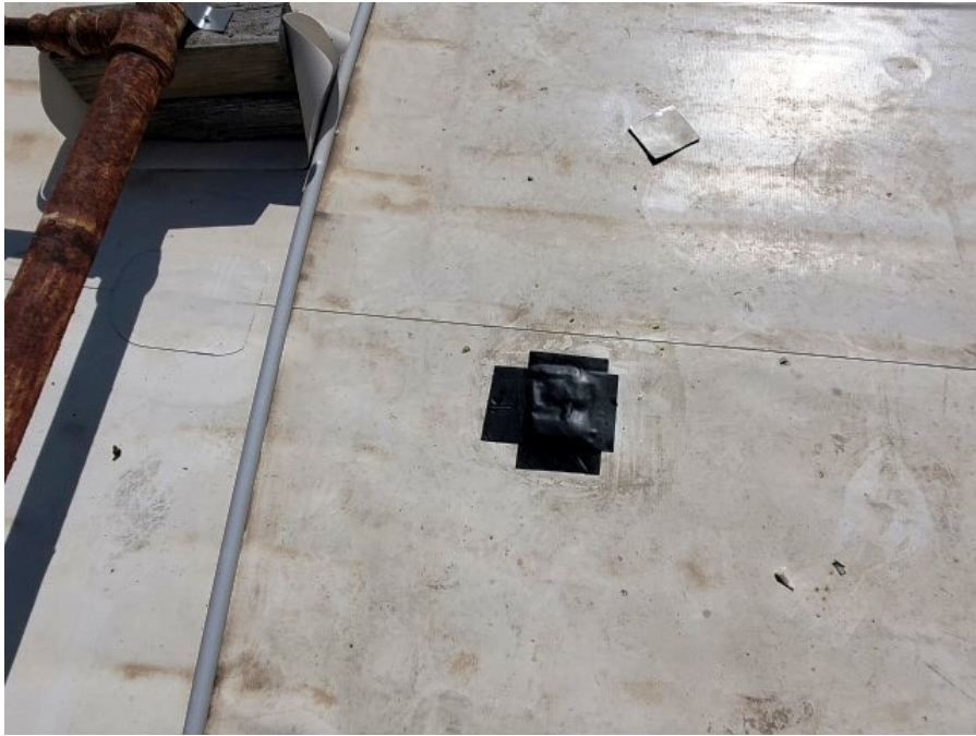
Photo 11: Temporary roof patch with primer adhesive.
