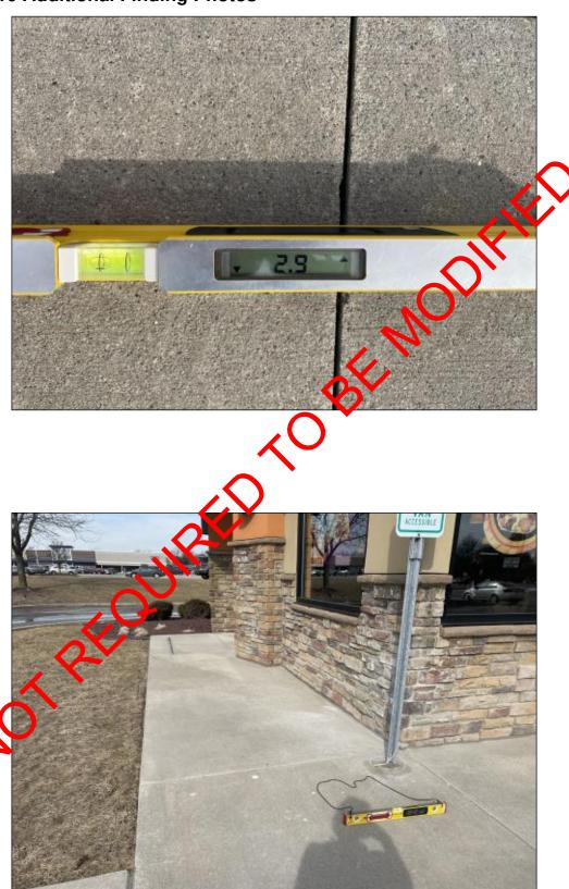
WITHIN REASONABLE CONSTRUCTION TOLERANCE
