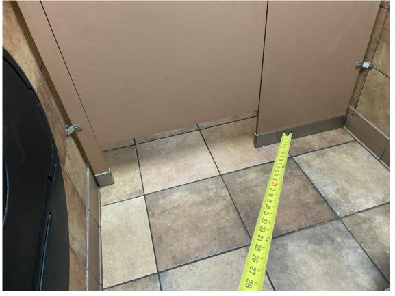
**NOTE:** IF THIS COMPARTMENT WAS ORIGINALLY CONSTRUCTED PRIOR TO MARCH 2010, IT CAN REMAIN AS-IS. OTHERWISE, THE COMPARTMENT WILL NEED TO BE MODIFIED TO CONFORM TO CURRENT ADA STANDARDS.
