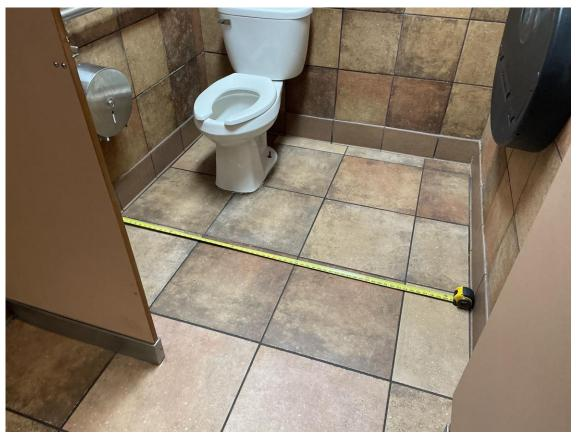
**<u>NOTE:</u>** IF THIS COMPARTMENT WAS ORIGINALLY CONSTRUCTED PRIOR TO MARCH 2010, IT CAN REMAIN AS-IS. OTHERWISE, THE COMPARTMENT WILL NEED TO BE MODIFIED TO CONFORM TO CURRENT ADA STANDARDS.
