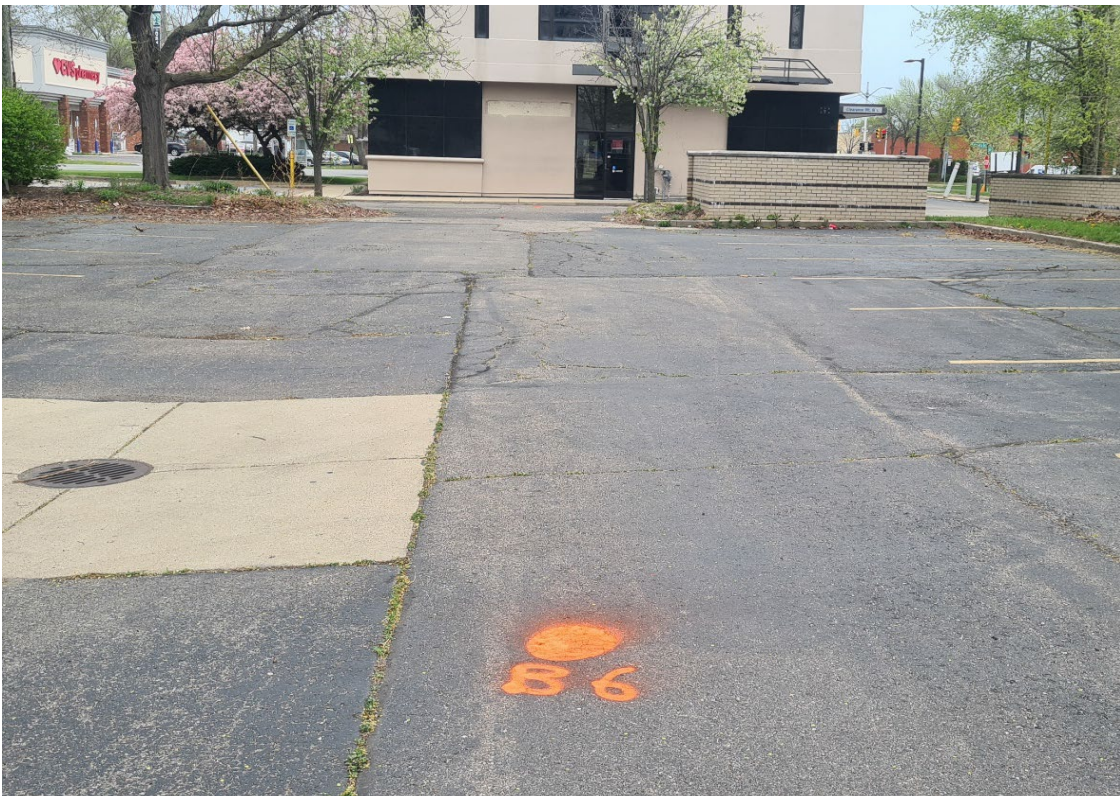
Photo No. 6 - From B-06 Facing Northeast
