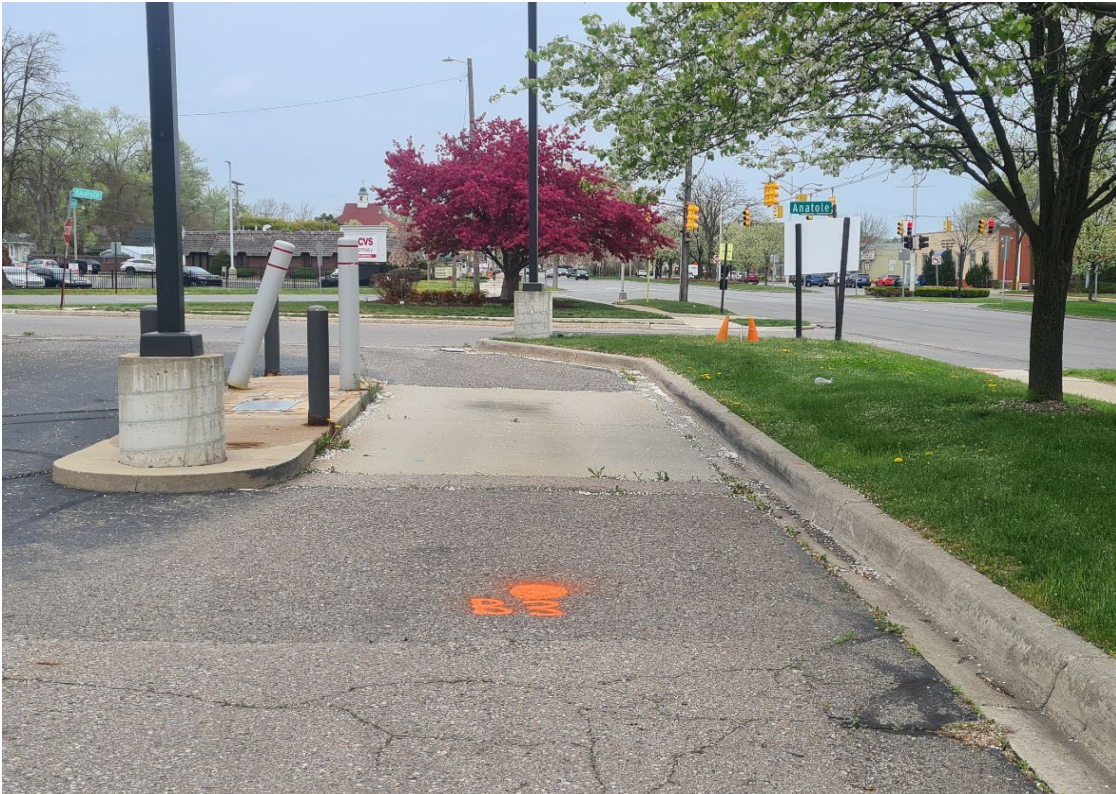
Photo No. 3 - From B-03 Facing Northeast
