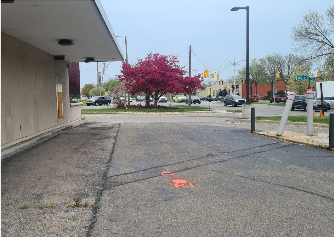
Photo No. 1 - From B-01 Facing Northeast
