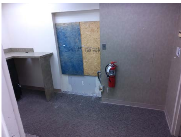
Drive Through Window Teller Area, 1st floor
