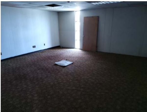
Office 003, 2nd Floor
