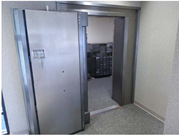
Vault, 1st floor
