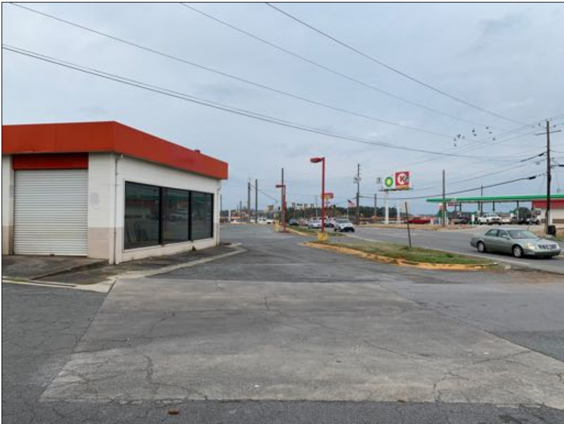
Looking west along the north side property line from northeast corner of the property
