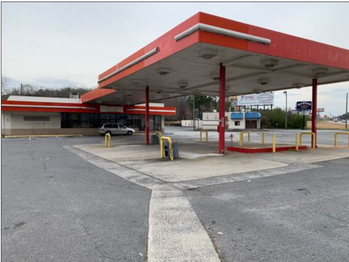
Looking south from the north property line at the fuel pump island and convenience store
