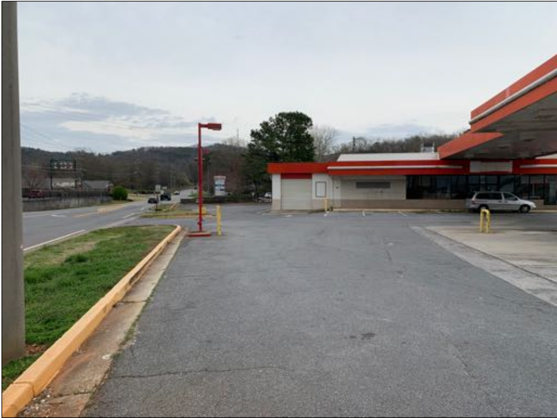
Looking east along the north side property line (E Felton Road)
