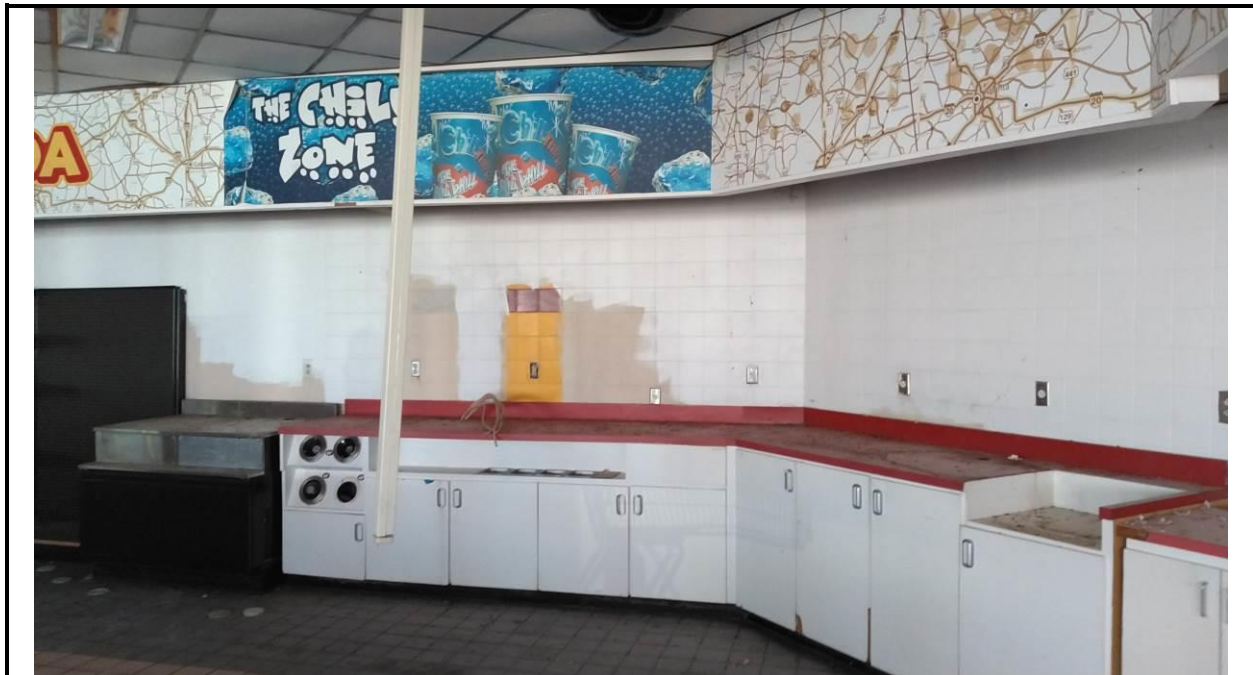
Photo 1: Non-ACM Drywall System (HSM 01)
