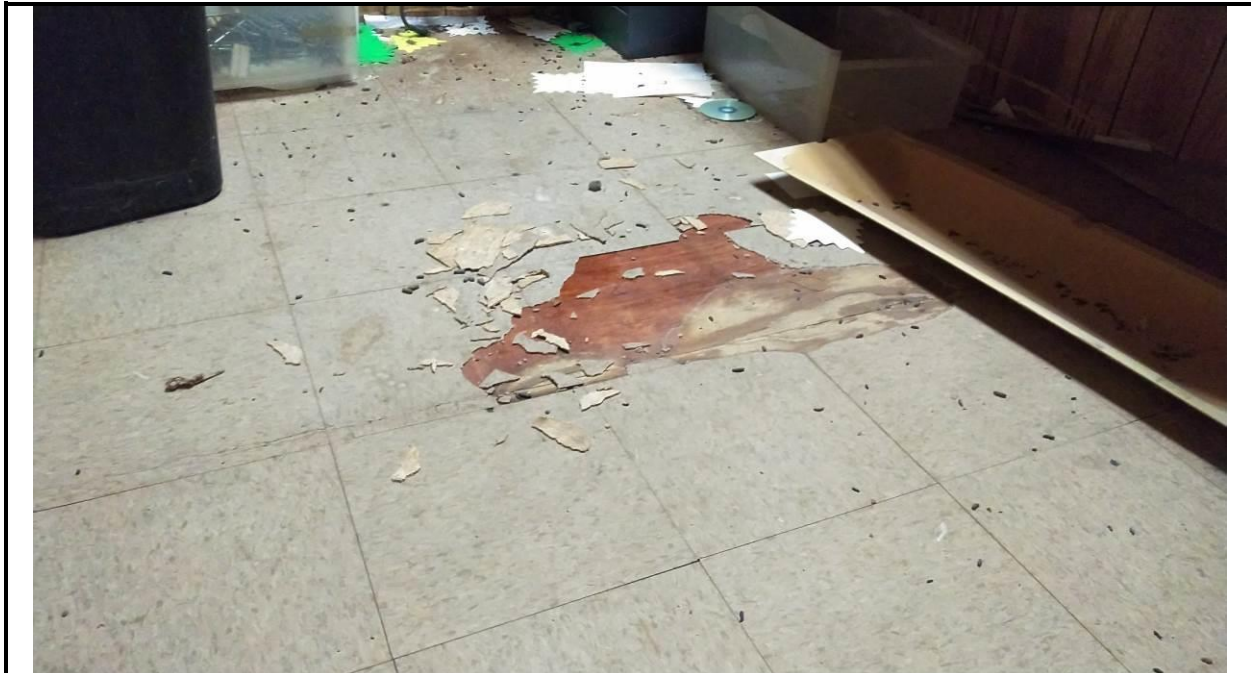
Photo 3: Non-ACM 12" X 12" Cream Colored Floor Tile and Mastic (HSM 03)
