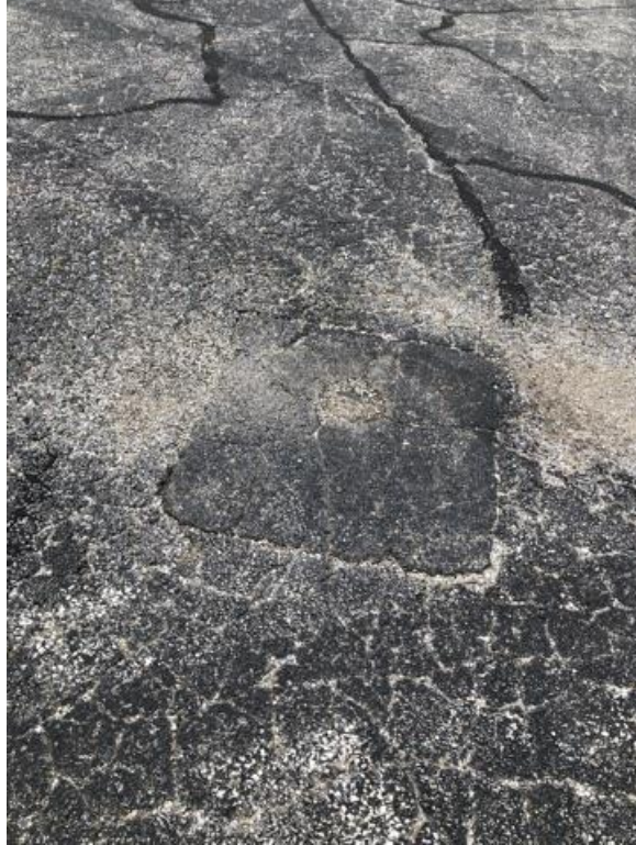
Photo 5: View of small manhole.
