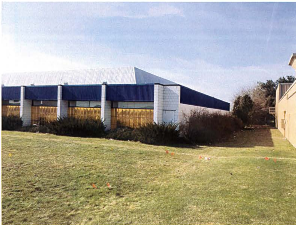
5603 Subject Property North Border as Viewed from the East
