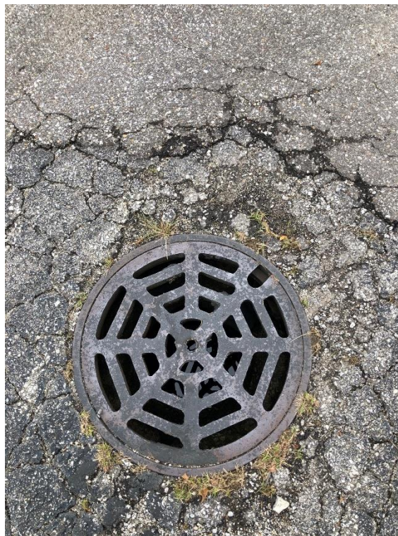
Photo 4: View of typical drain.
