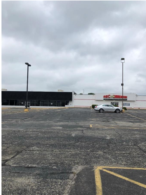
Photo 2: View of west adjacent properties.
