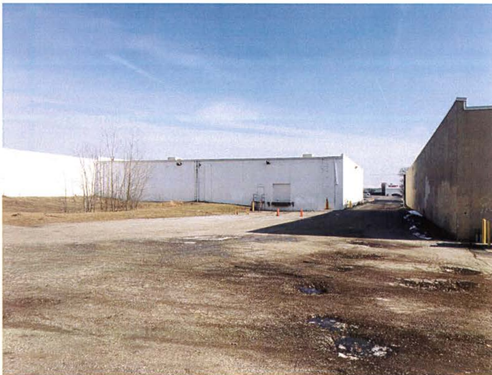
5505 Subject Property as Viewed from the West
