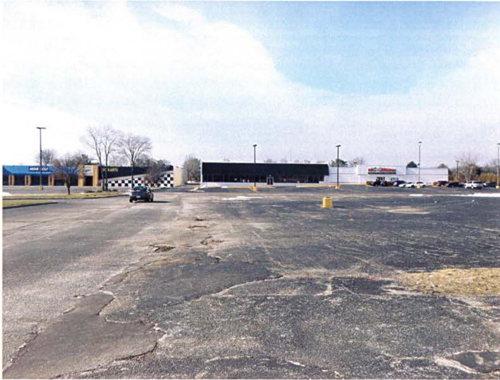
5505 Subject Property as Viewed from the East
