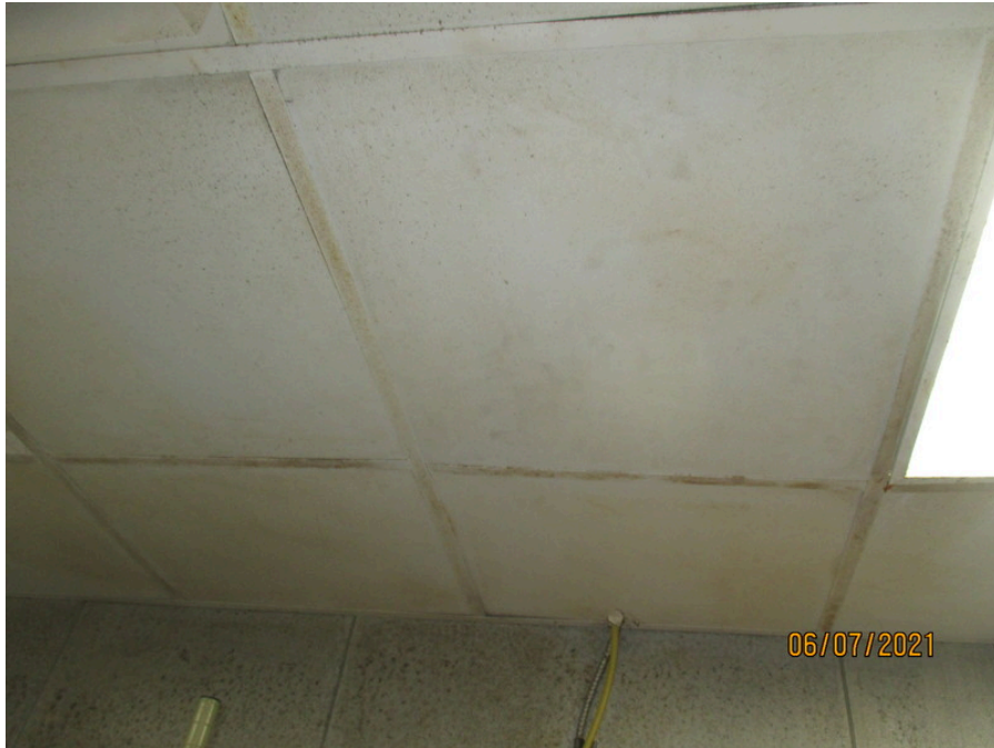
Photo 5: Non-asbestos containing gypsum board ceiling tile, observed and sampled in the kitchen (5A-5C)
