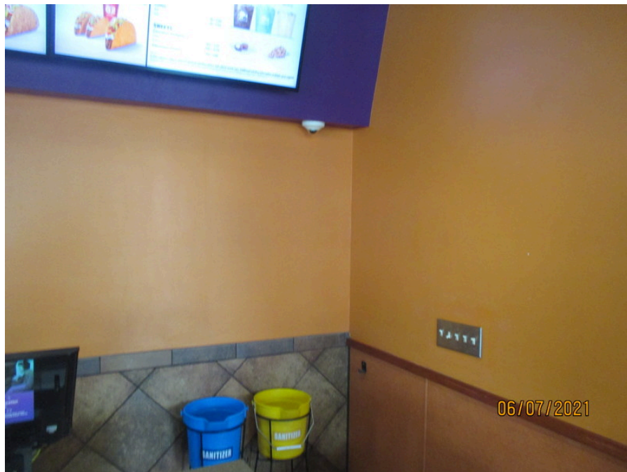
Photo 2: Non-asbestos containing drywall and joint compound, observed and sampled in the dining room (2A-2C)
