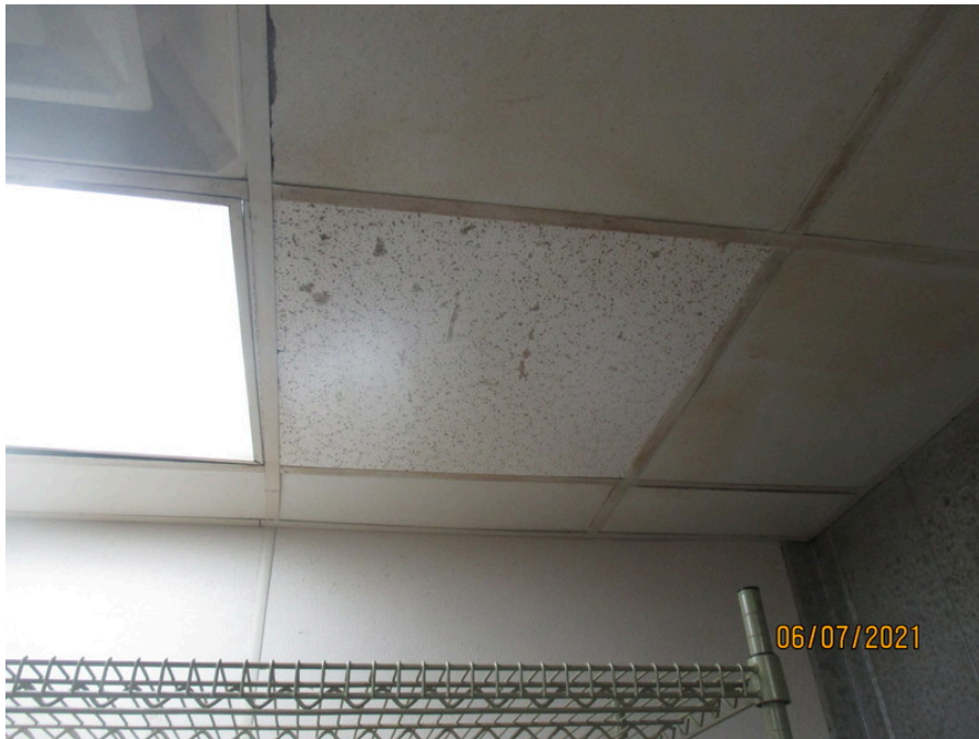
Photo 6: Non-asbestos containing ceiling tile, observed and sampled in the kitchen (6A-6C)
