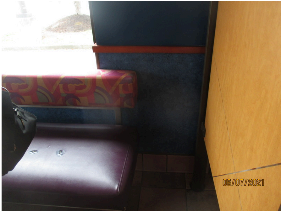
Photo 4: Non-asbestos containing blue lower wall covering, observed and sampled in the dining room (4A-4C)
