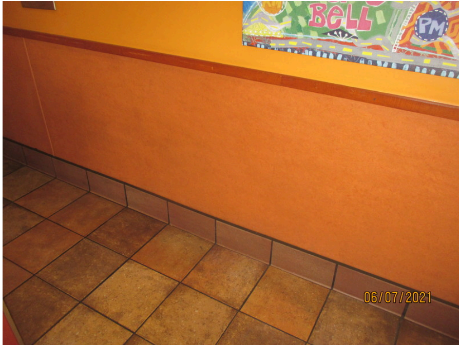
Photo 3: Non-asbestos containing orange lower wall covering, observed and sampled in the dining room (3A-3C)
