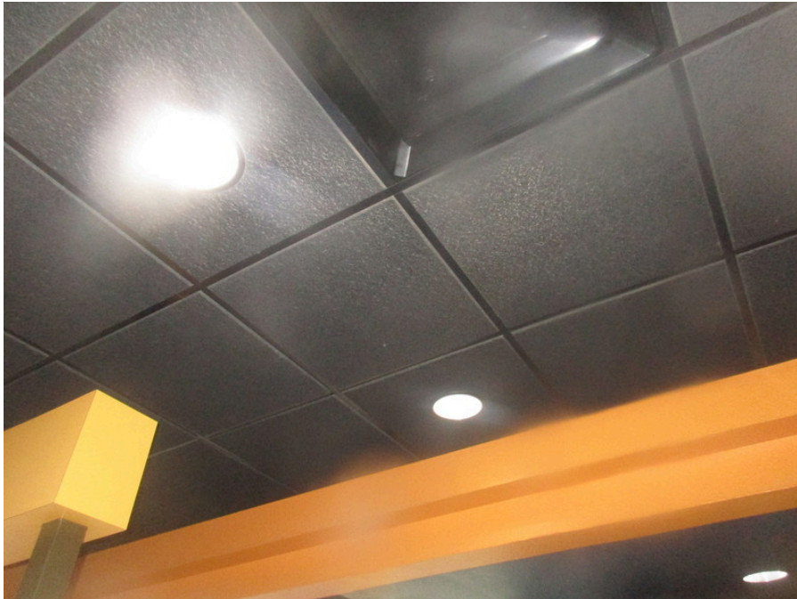
Photo 2: Black ceiling tile
