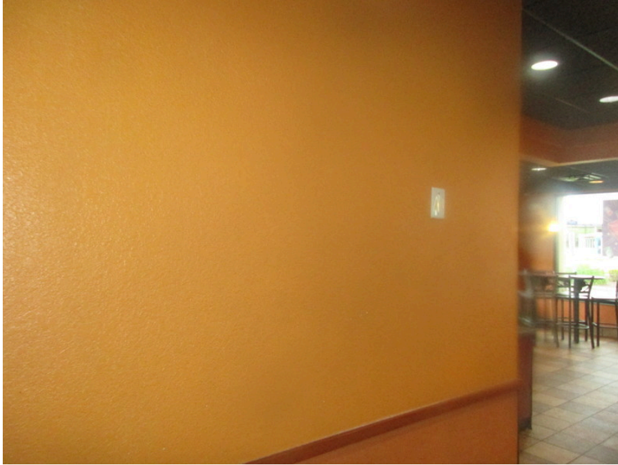
Photo 1: Drywall and skim coat
