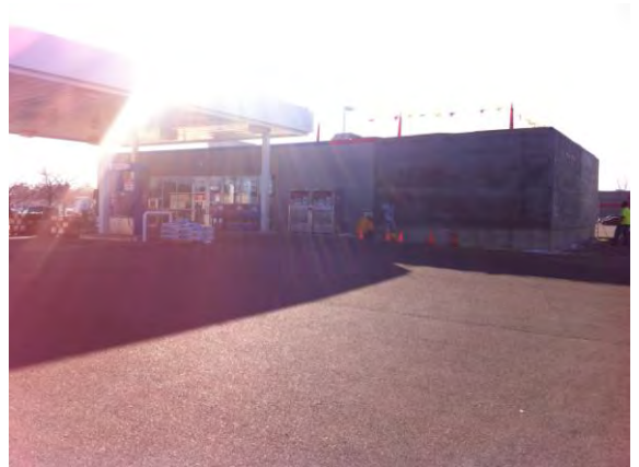
Photo #10: View of west adjoining filling station property
